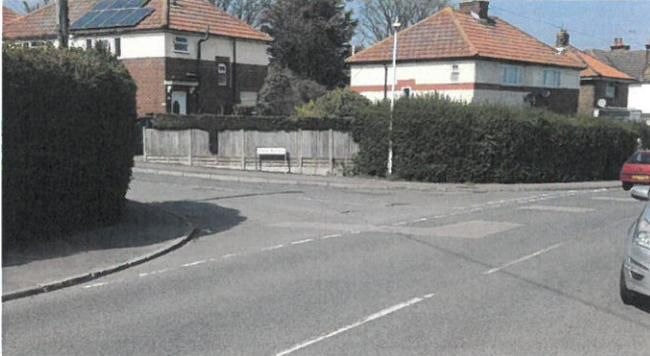
Path outside Mill Inn on Mill Hill - Camber of path by bus stop causes wheelchair and scooter to drift severely towards the road.
