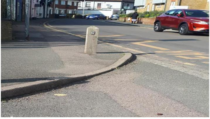
4. Golf road turning onto Harold Road, the drop kerb is slightly raised making it extremely difficult to use for a wheelchair or buggy user.
