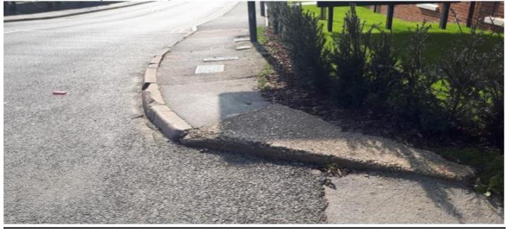
2. No drop kerb to allow safe crossing leading to houses 71-81 of Golf Road. Drop kerbs were present on the other side (Athelstan Place) but to use these would require crossing the road using dropped driveways that are not adequate.
