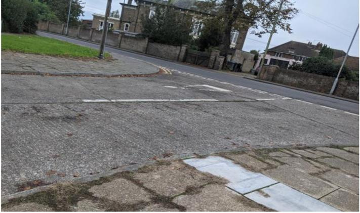
7. Coming down London Road from St Leonard's Church on the right-hand side, the pavement has areas badly in need of repair, some slabs were uneven and cracked which is a safety issue for pedestrians unsteady of their feet and for wheelchair and buggy users.
