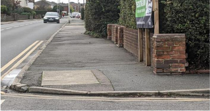
4. Walking from town on the right-hand side of London Road going towards the hospital, there were several areas of badly cracked and uneven paving slabs, which are trip hazards and dangerous for the visually impaired.
